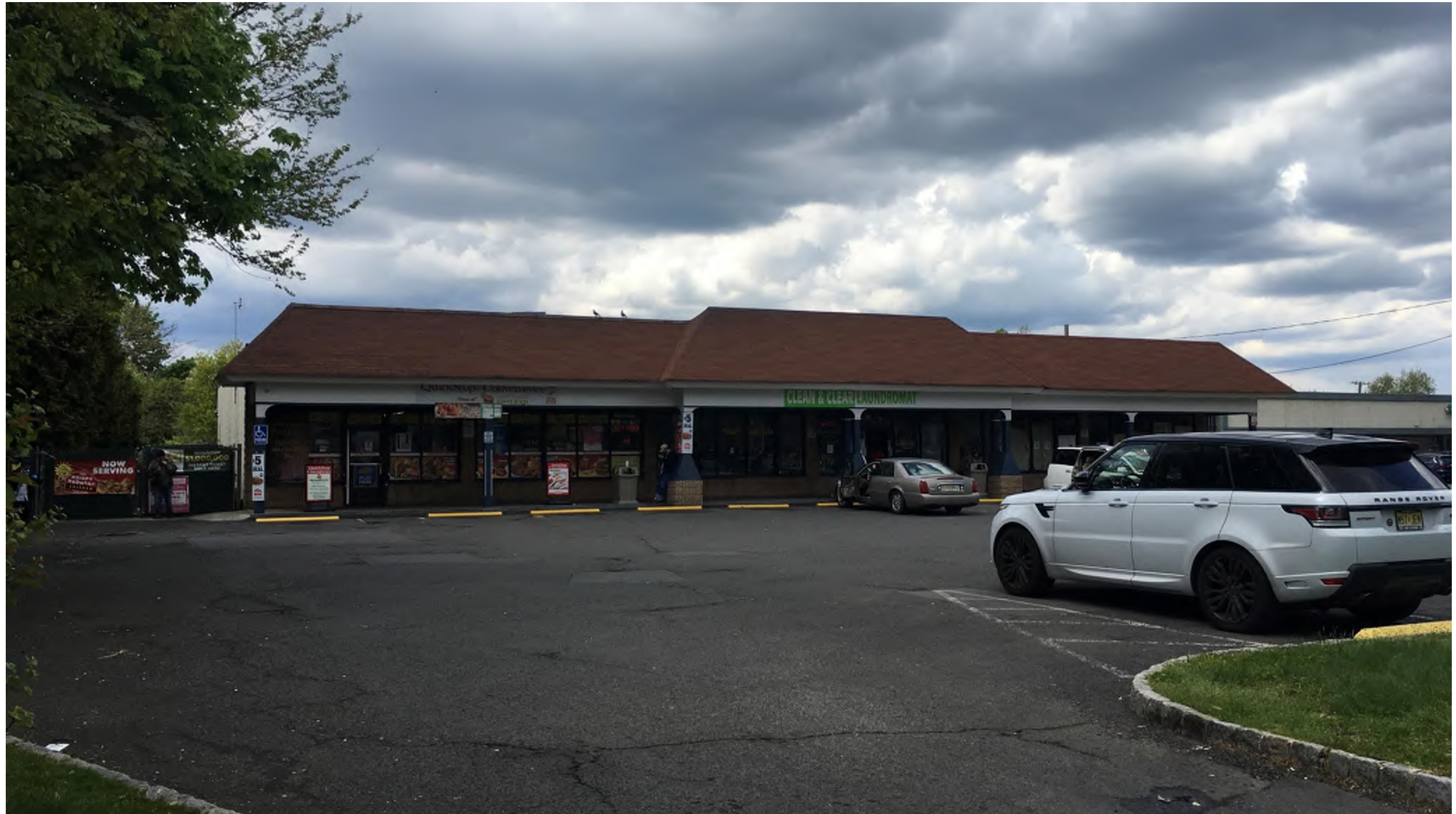
VIEW OF THE EASTERN FAÇADE OF EXISTING BUILDING, WHICH FACES WEST 7 TH STREET, WITH SURFACE PARKING IN FRONT (TAKEN MAY 12, 2020)
